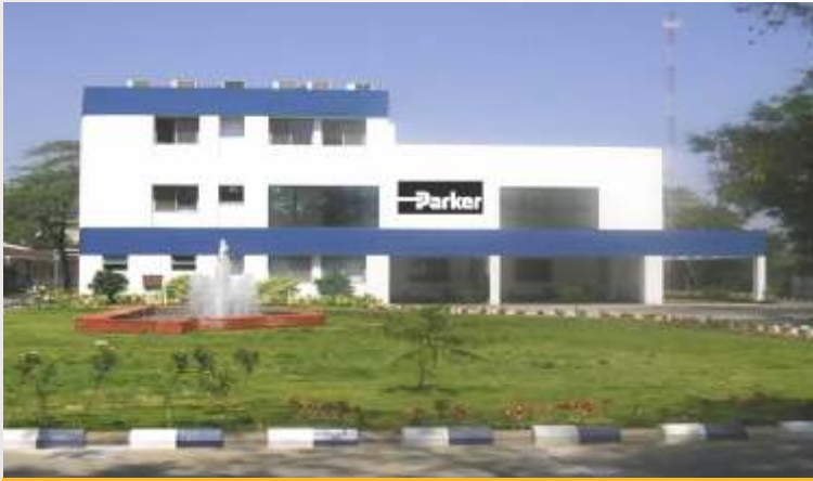
Hose & Fittings Plant, Hyderabad
