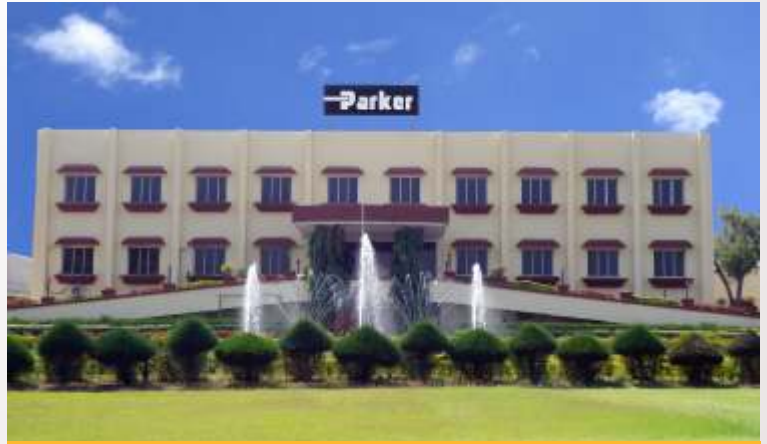
Hose Plant, Nagpur
